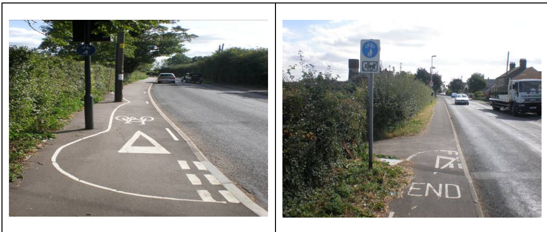
Figure 3-5: Rampton Rd Dedicated Cycle Lane
